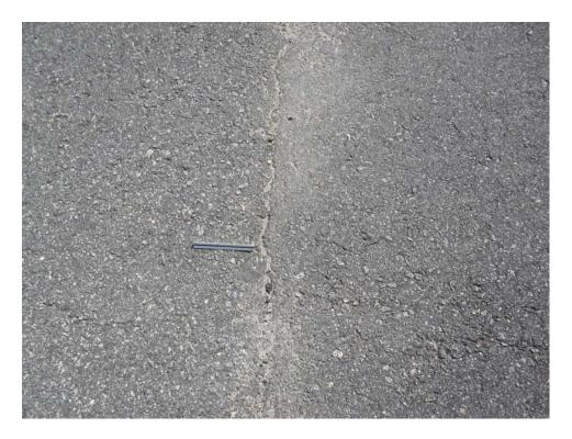
A01MR-70. Longitudinal and Transverse Cracking.
