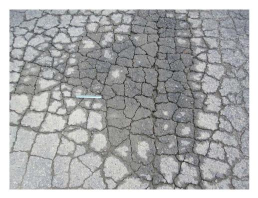
A01MR-10. Alligator Cracking (Sample Unit #01).
