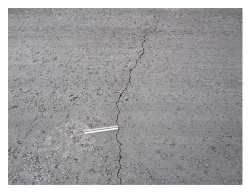
TAMR-20. Longitudinal and Transverse Cracking (Sample Unit #01).
