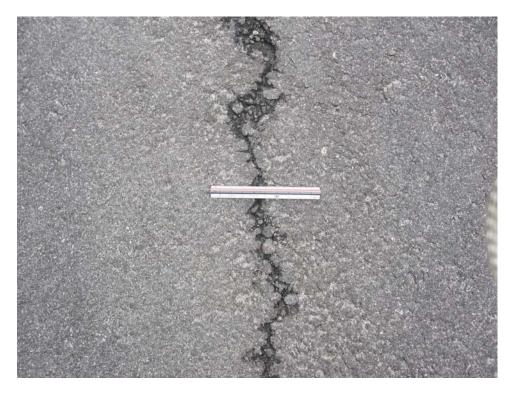
A01MR-50. Longitudinal and Transverse Cracking (Sample Unit #12).
