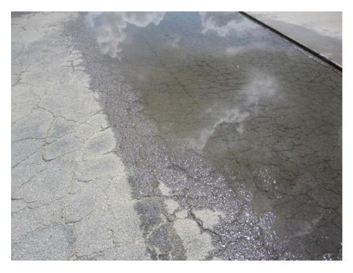
A01MR-60. Rutting and Alligator Cracking (Additional Sample Unit #01).
