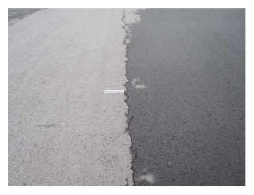
A02MR-10. Longitudinal and Transverse Cracking.
