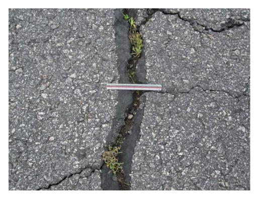
A03MR-10. Longitudinal and Transverse Cracking (Sample Unit #14).
