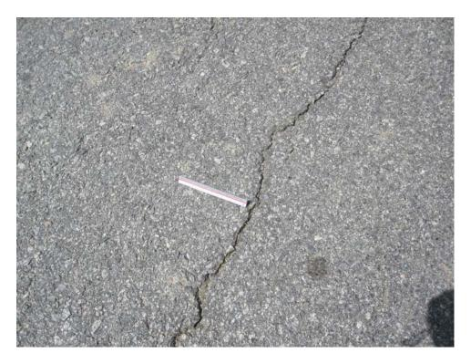
A01MR-60. Longitudinal and Transverse Cracking (Sample Unit #03).
