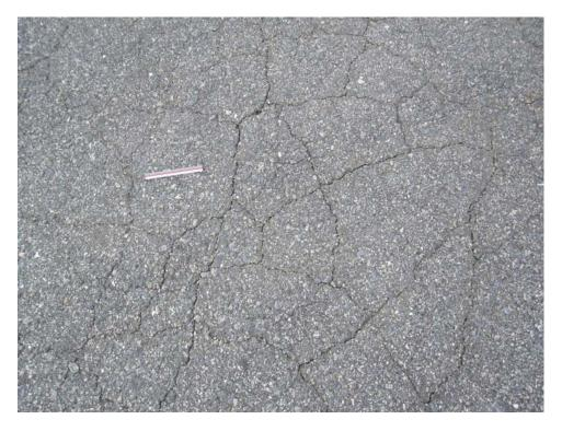
A01MR-40. Alligator Cracking (Sample Unit #56).
