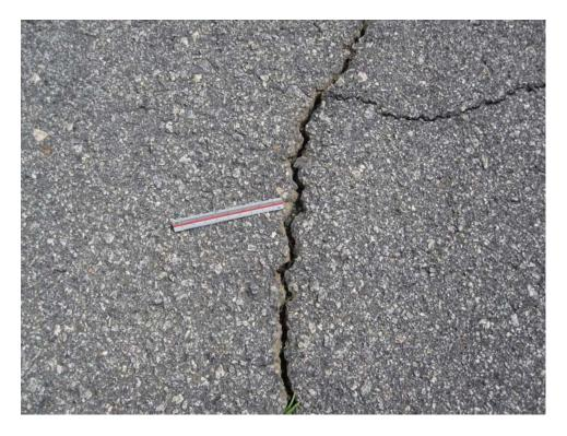
A01MR-40. Longitudinal and Transverse Cracking (Sample Unit #10).
