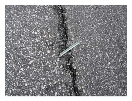
TBMR-10. Longitudinal and Transverse Cracking (Sample Unit #17).
