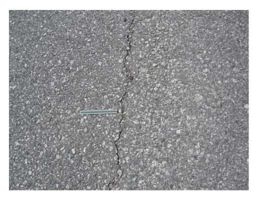
A01MR-20. Longitudinal and Transverse Cracking (Sample Unit #03).
