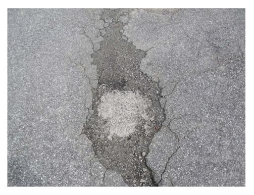
A01MR-10. Alligator Cracking (Sample Unit #04).
