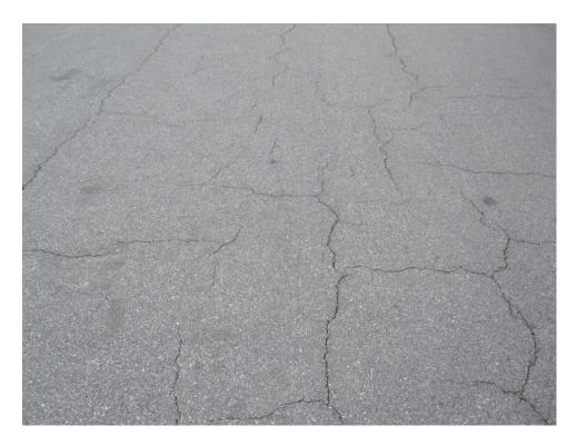
A01MR-30. Block Cracking (Sample Unit #04).
